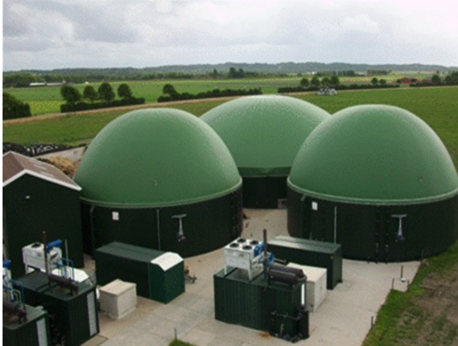
Figure 21: Decentralized Bio-fermentation Plant
